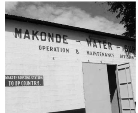
Water Supply Booster Station
