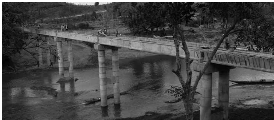
Bridge in Project Area
