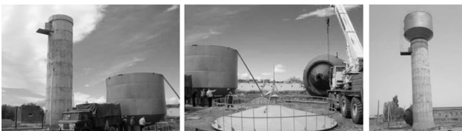
Assembling new steel tank on site
