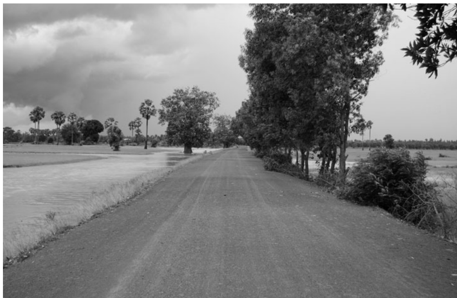
Laterite road rehabilitated under Tertiary Road Improvement Programme IV in Prasat Sambo District
