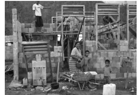
Reconstruction of houses
