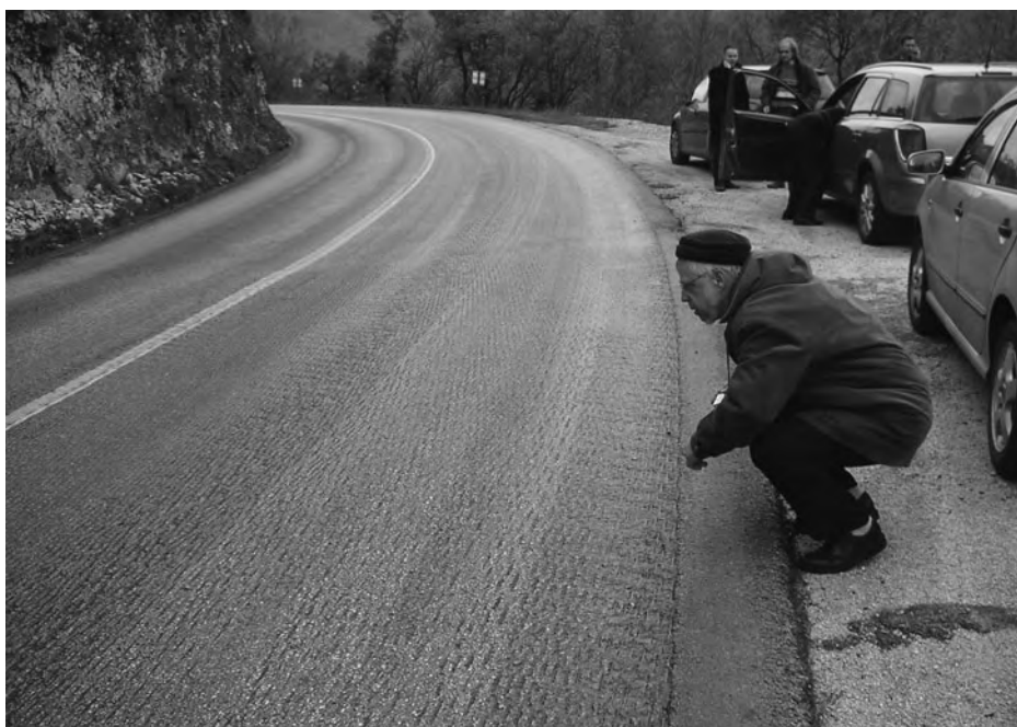
Road inspection during field visit in Istria
