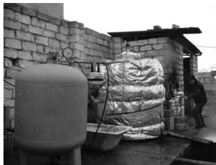
Small Scale Biogas facility (3m 3 Digester)
