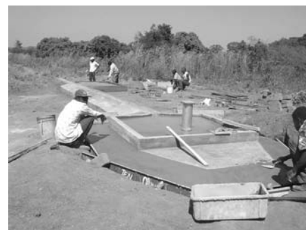
Construction of Civil Works
