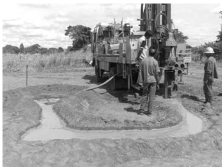
Drilling (Mud-rotary method)
