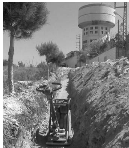
Passing Sewer pipes in the Village Tefahta
