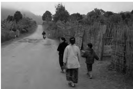
Lao PDR: View of RN6 section to be rehabilitated
