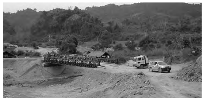
Lao PDR: Bridge construction in Bokeo
