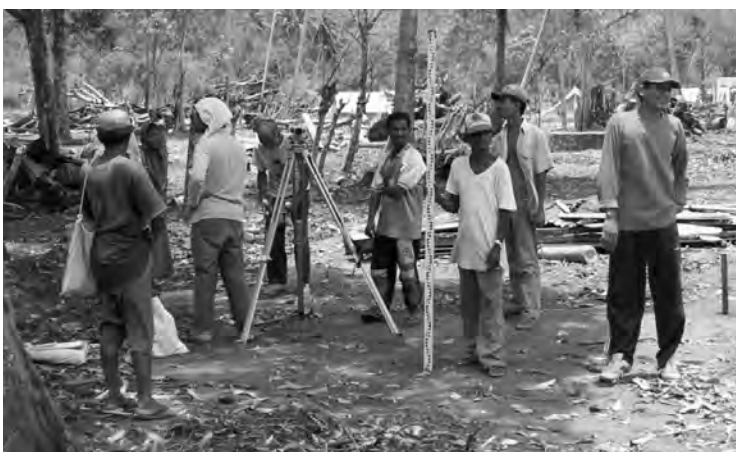
Indonesia: Survey Works in Progress
