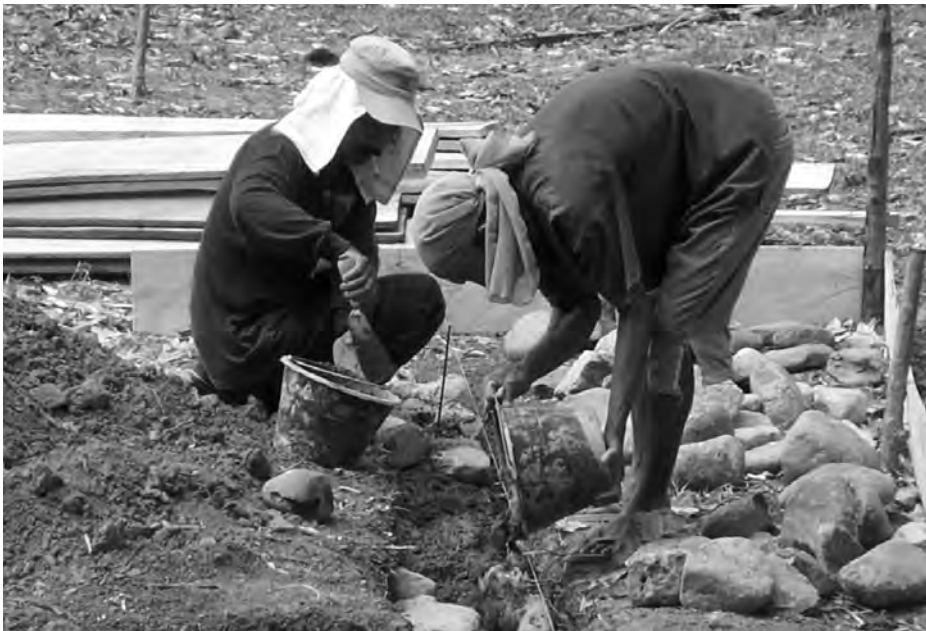
Indonesia: Foundation Works
