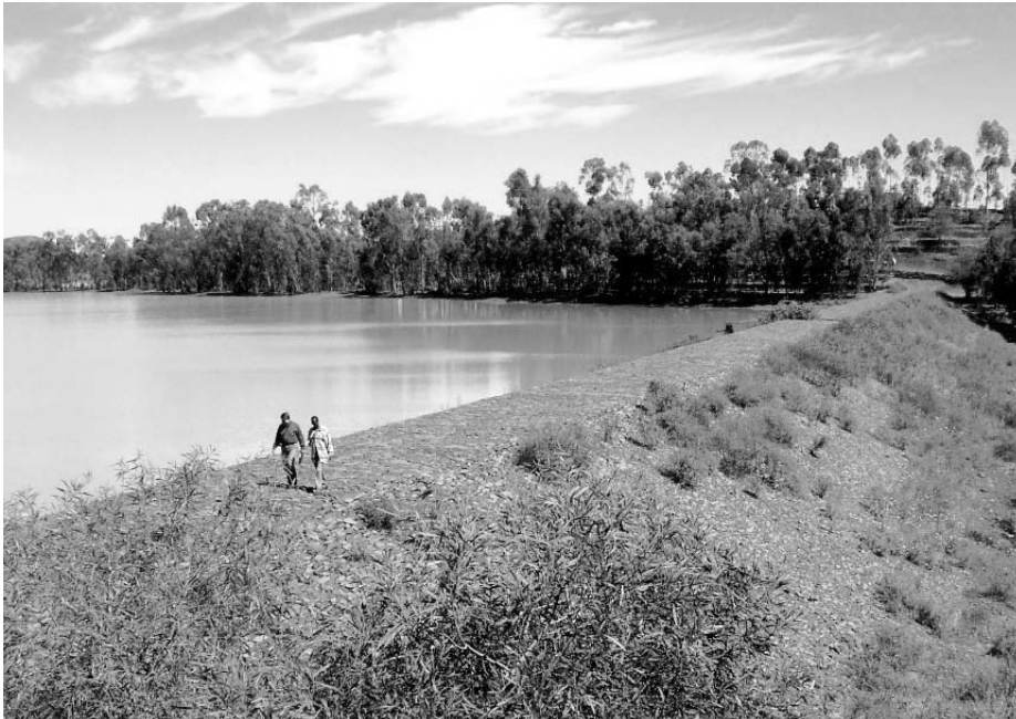
Eritrea: Kilwale dam stone protection
