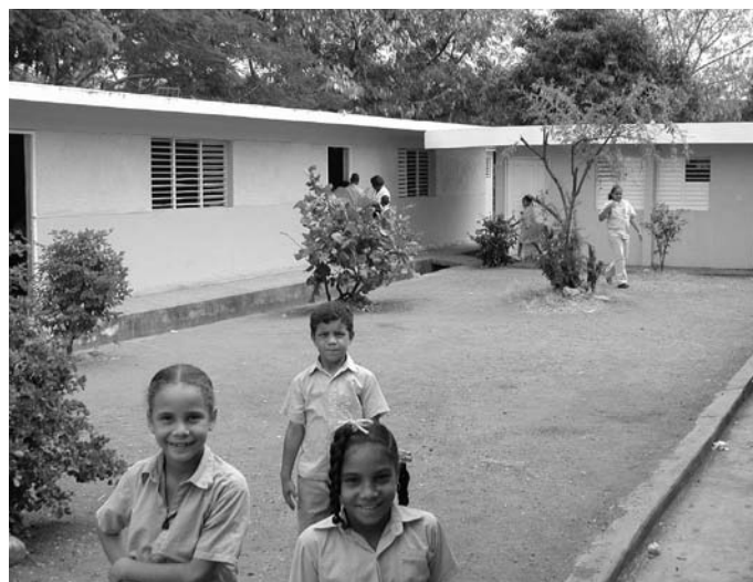
DOMINICAN REPUBLIC: Newly constructed typical Primary School
