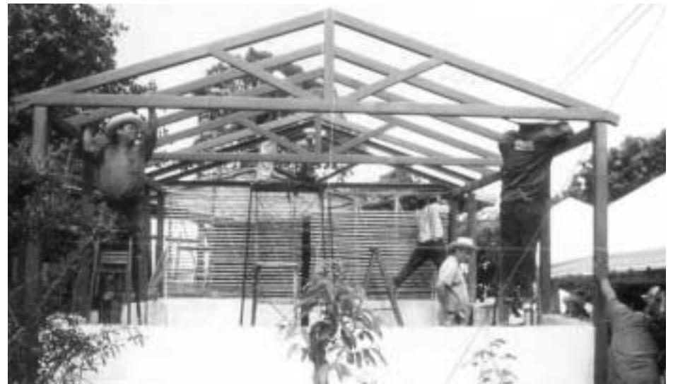
EL SALVADOR: Construction of a Standard House with Steel Structure
