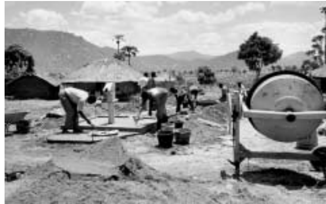
MALAWI: Concrete Works for a Well Apron
