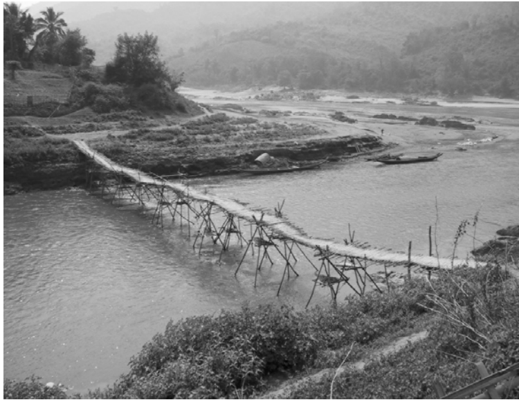
LAO PDR: Temporary River Crossing over the Nam Tha
