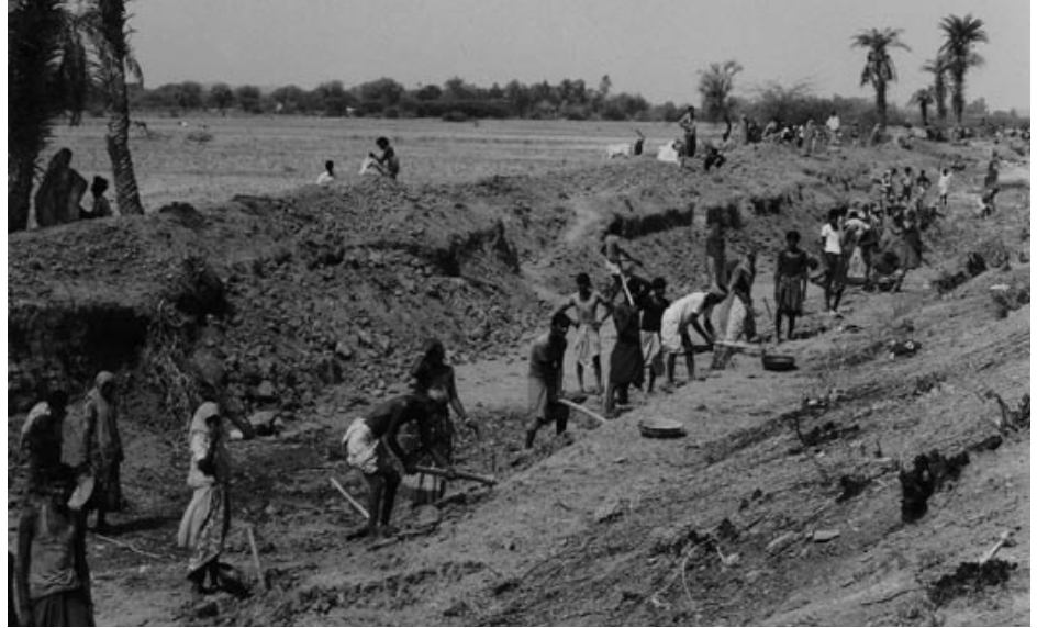
INDIA: Participation of Water Users in Rehabilitation of an Irrigation Main Canal (Famine Relief Work)
