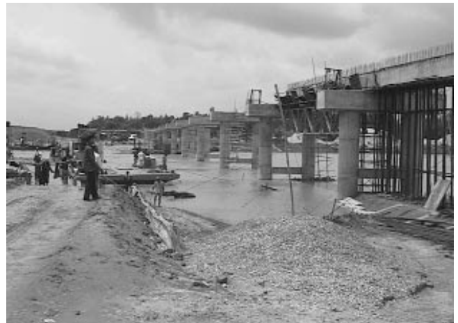
BANGLADESH: Construction of the Hatubhanga Bridge
