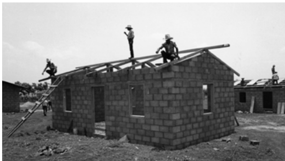
HONDURAS: Setting-up of a Roof Structure for a Low-cost House
