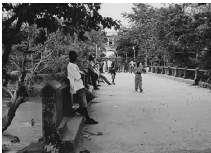
HAITI: Existing Bridge over the Massacre River
